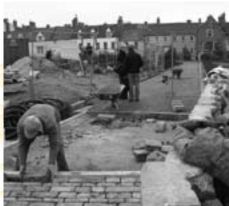
■ Work in progress on the new perimeter road
