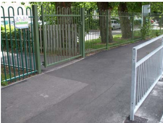
Infant school safety rail and re-surfacing
