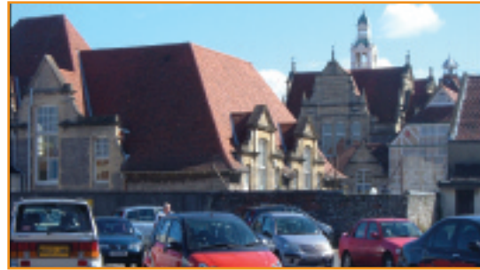
Photo No.6 – The Carlton Centre and Walliscote Primary School
